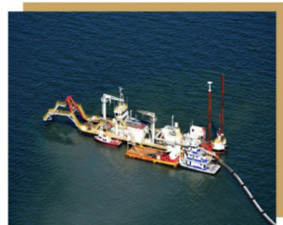
Manson Construction – Robert M. White Cuttersuction Dredge (30-Inch) Halimar Shipyard, LA - $40 M. (Delivered, in service 2018)
