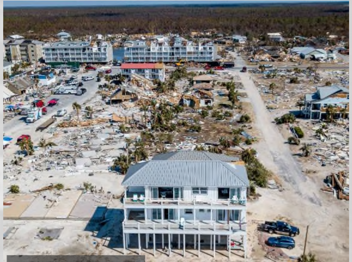
Hurricane Michael Mexico Beach, FL (October 2018)
