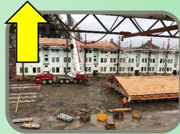
DA MILCON and Installation Support $8.4B / 3 million service men and women / 287 Installations
