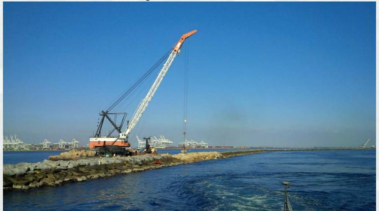
• Breakwater repair is on-going. Connolly Pacific completed three breached areas and rebuilt the head of San Pedro Breakwater.
