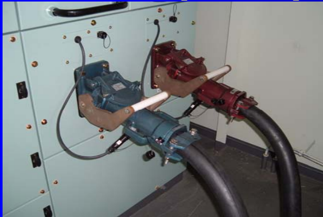
Shore connection panel on ship
