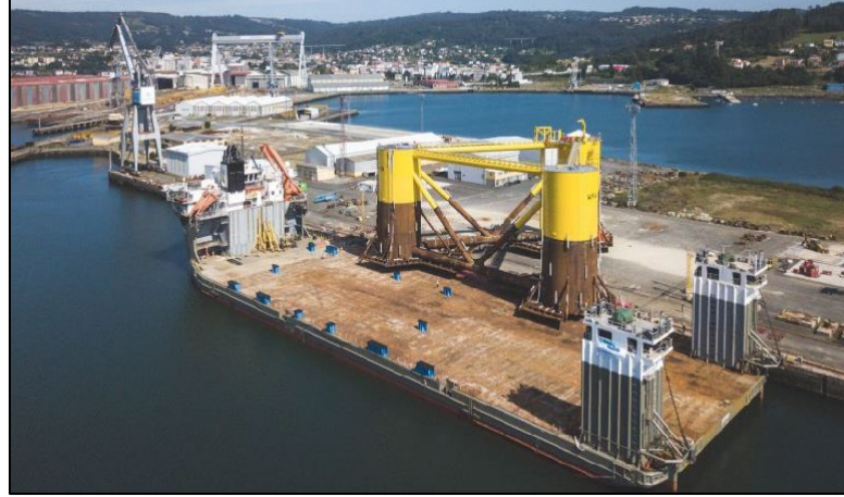
2) Loadout onto semi sub
