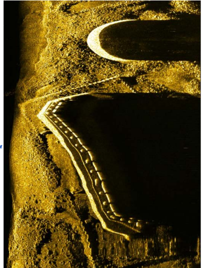
Bridge footing (Jacksonville, FL)
