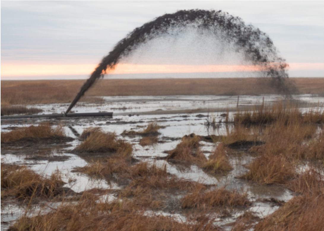
Thin layer placement of dredged sediment (source: https://usfwsnortheast.wordpress.com/2017/08/16/a-bottom-up-boost-for-coastal-habitat/ )
