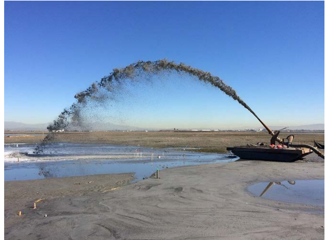
Seal Beach thin layer placement (source: US Army Engineer and Research Development Center)
