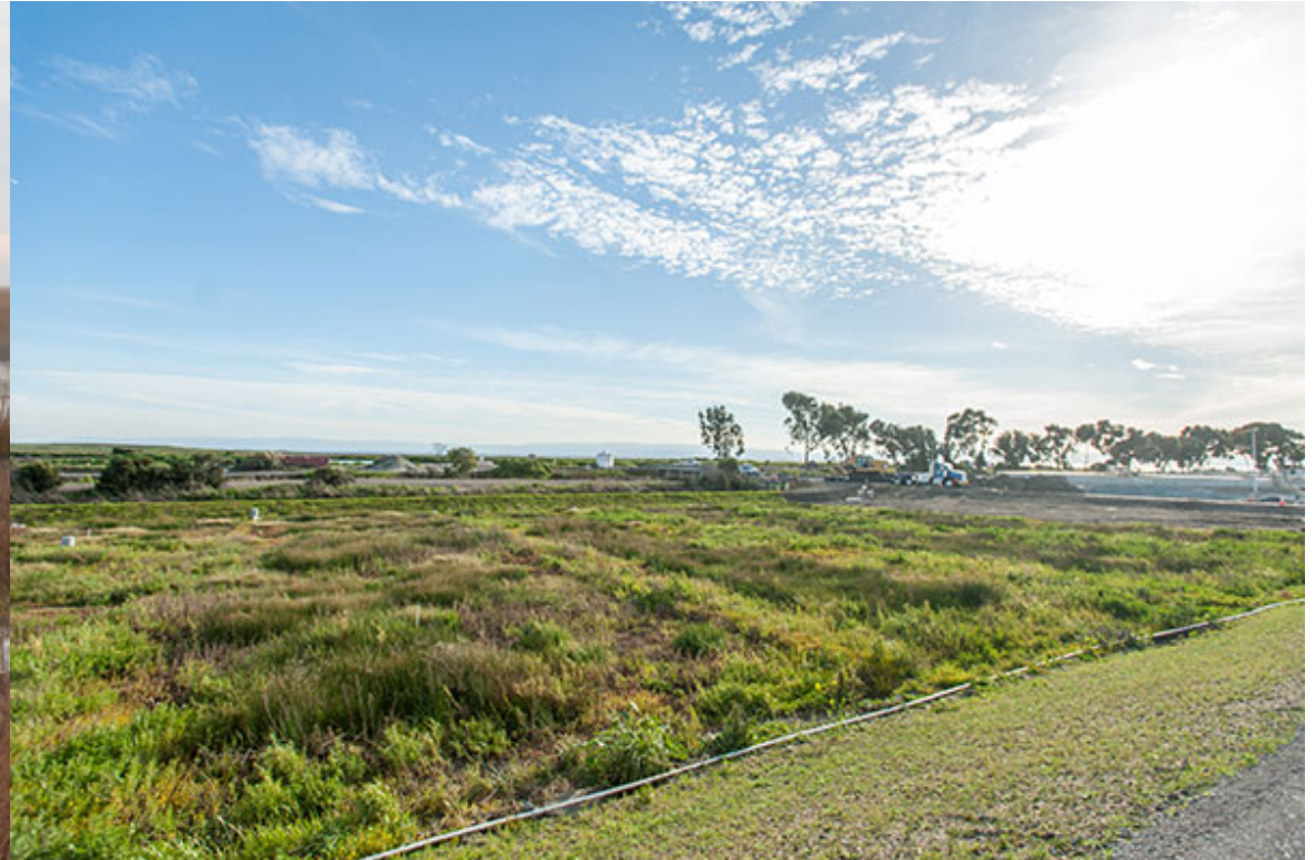
Oro Loma horizontal levee. (source: https://oroloma.org/horizontal-levee-is-thriving/ )
